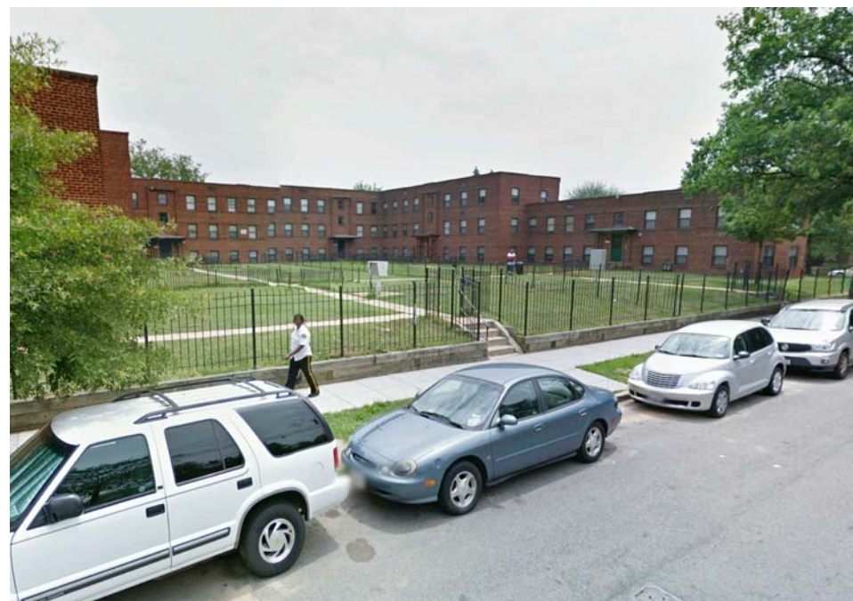
ADJACENT PROPERTY (SOUTH)
